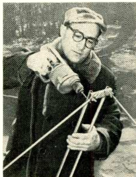
Fig. 1—Drilling in terminal block.
