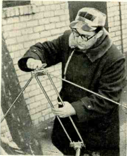
Fig. 2—Tapping the drilled hole.
